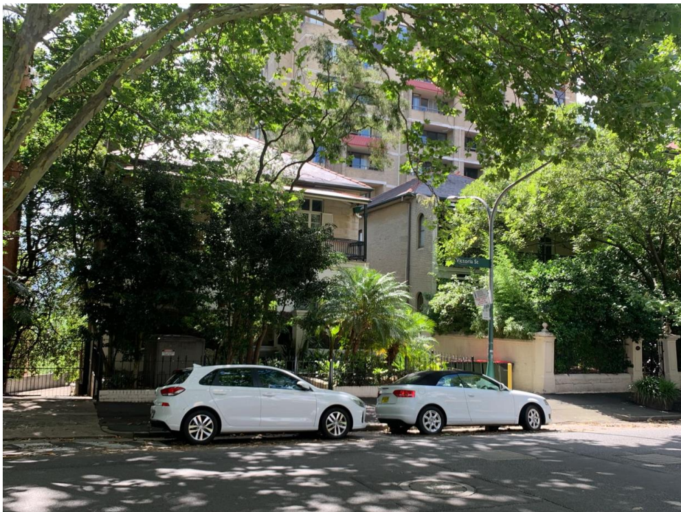
Figure 4: Adjoining heritage items to the northeast at 101-115 Victoria Street, viewed from Victoria Street
