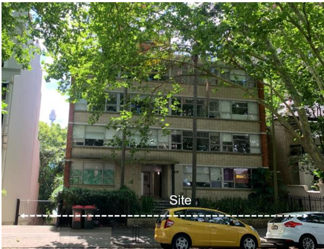
Figure 2: Site viewed from Victoria Street, looking west
