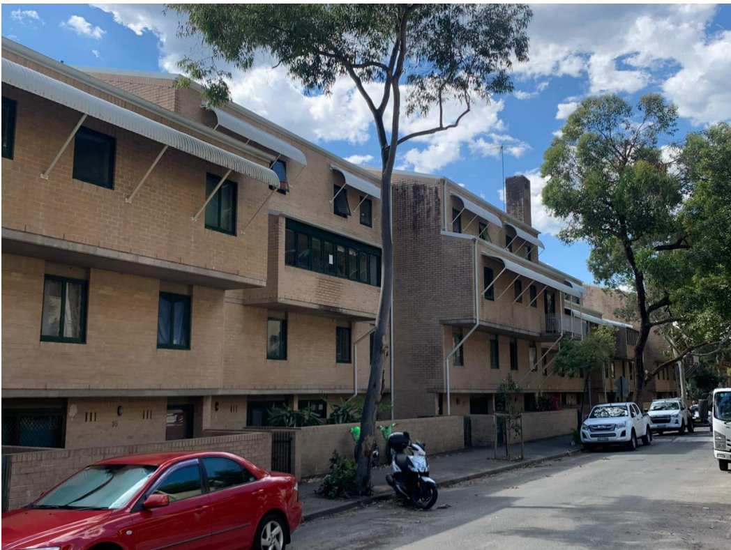
Figure 8: Buildings to the west across Brougham Street at 79-85 Brougham Street, viewed from Brougham Street
