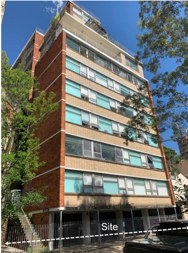
Figure 3: Site viewed from Brougham Street, looking east
